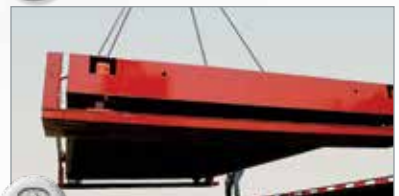
2 Unload and set modules.
