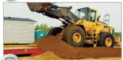
3 Backfill to bulkheads and finish ramps.
